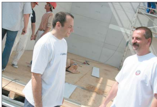
The mobile squash court under construction.
